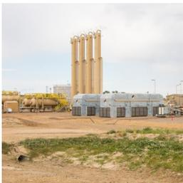
**Pipelines and Gathering Facilities:** Crestone utilizes pipelines and central gathering facilities to minimize the footprint of well pads, helping reduce truck traffic and eliminating storage tanks and emissions sources. These facilities allow for use of more efficient emissions reduction techniques like floating roof tanks and chillers.
